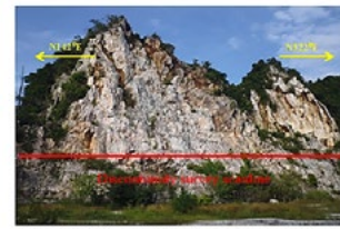
Figure 4: Slope GL2, Gunung Lang, Ipoh, Perak, Malaysia.
