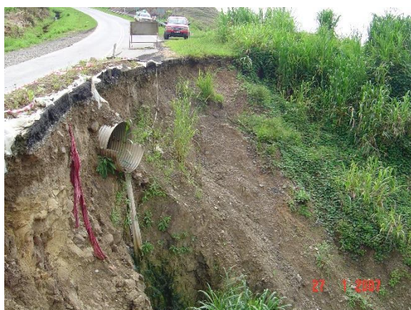
Figure 4: Embankment failure in the form of a deep slide (T1 – b) at KM 45 (SS6)
