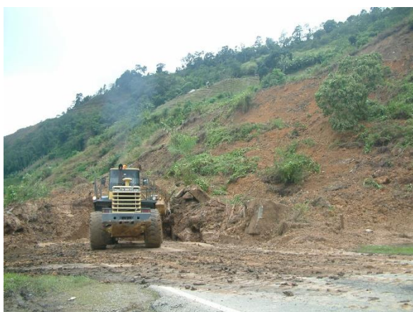
Figure 4: Embankment failure in the form of a deep slide (T1 – b) at KM 45 (SS6)
