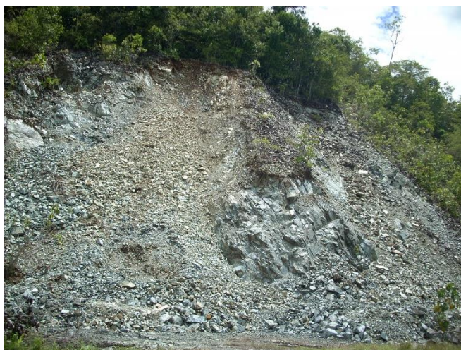
Figure 7: Circular failure (crushed) (B1 – b) at East KM 21 (RS1) shows the surface weakness (revealing) within the structure, which composed of coherent crushed rocks on the gently sloping discontinuities
