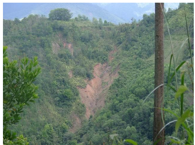
Figure 8: Wedge failure (blocks and fragments) (B3 – a) at KM 29 (RS2) indicates the form of discontinuities provides intersecting sheets to form yield stepped surfaces or boundary vertical joints
