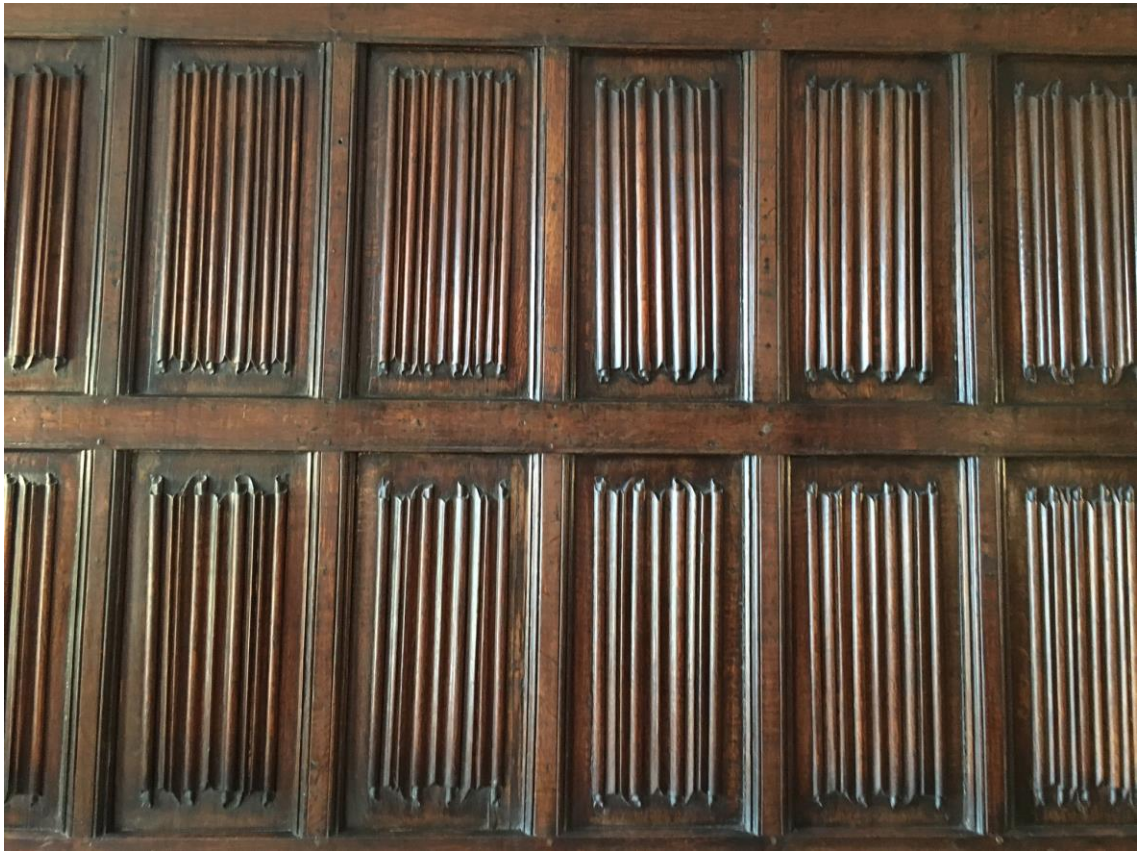
Figure 4.2 Detail of the Linenfold panels
