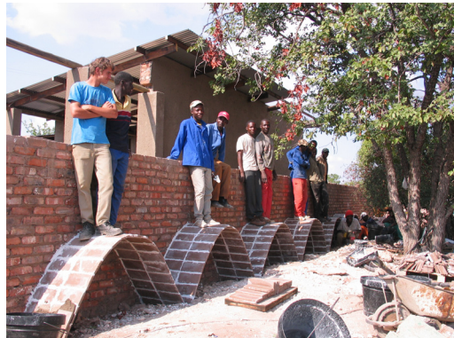
Figure 9: Test Vaults built on site
