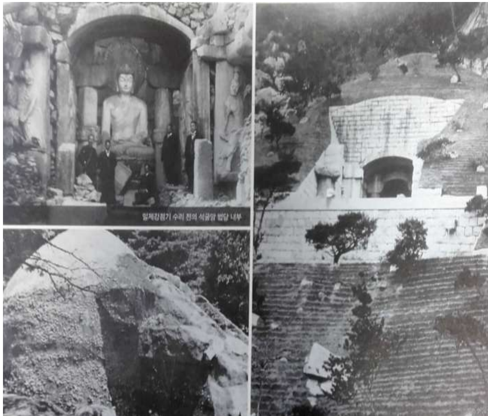
Fig 5.15 – Top left: The Seokguram grotto before Japanese intervention; Bottom left: The Seokguram Grotto during Japanese intervention when concrete was placed all around; Bottom right: The Seokguram Grotto in 1915 after the Japanese placed concrete all around the grotto (CHA 2011:77).
