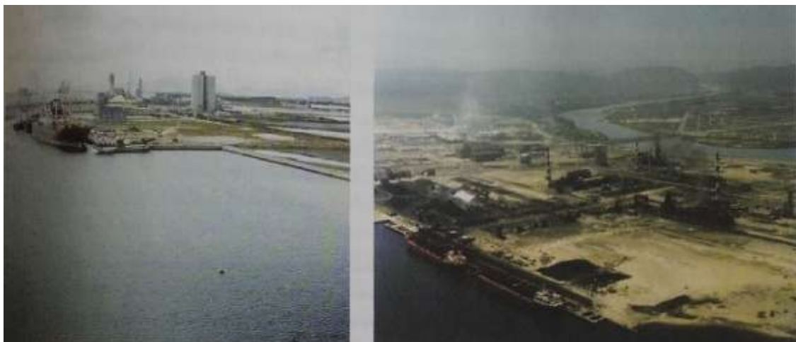
Fig. 3.9 Photographs of the Ulsan Industrial Complex and Ulsan Seaport (right) and the Pohang Iron and Steel Company (left) (Sakong and Koh 2013:179)
