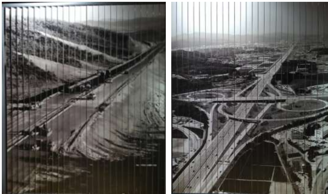
Fig. 3.7 Iconic blinds showing of the Seoul-Busan expressway during (left) and after (right) construction (both images are from the display at the National Museum of Korean Contemporary History)
