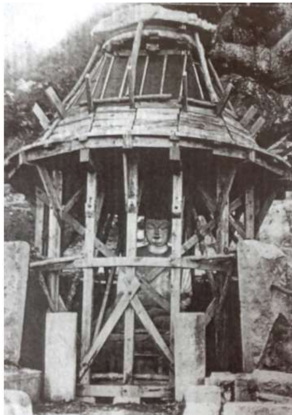
Fig 5.14 - The Grotto before repair works in 1915 (CHA 2009:181)
