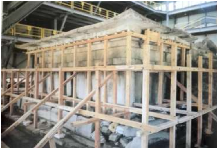
Fig.6.11 The rebuilding project in 2009 – laying down the first floor (CHA 2009:174)
