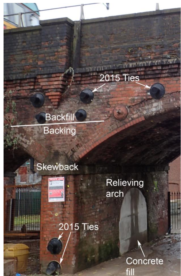
Figure 4. Northern view of the pier between Arches 38 and 39.
