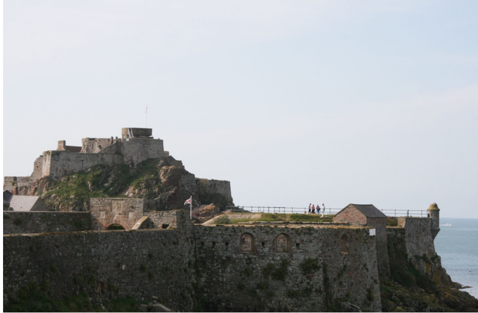
Fig.7 Elizabeth Castle installation site for Variable 4 . Elizabeth Castle, Jersey, 24 September 2011.
