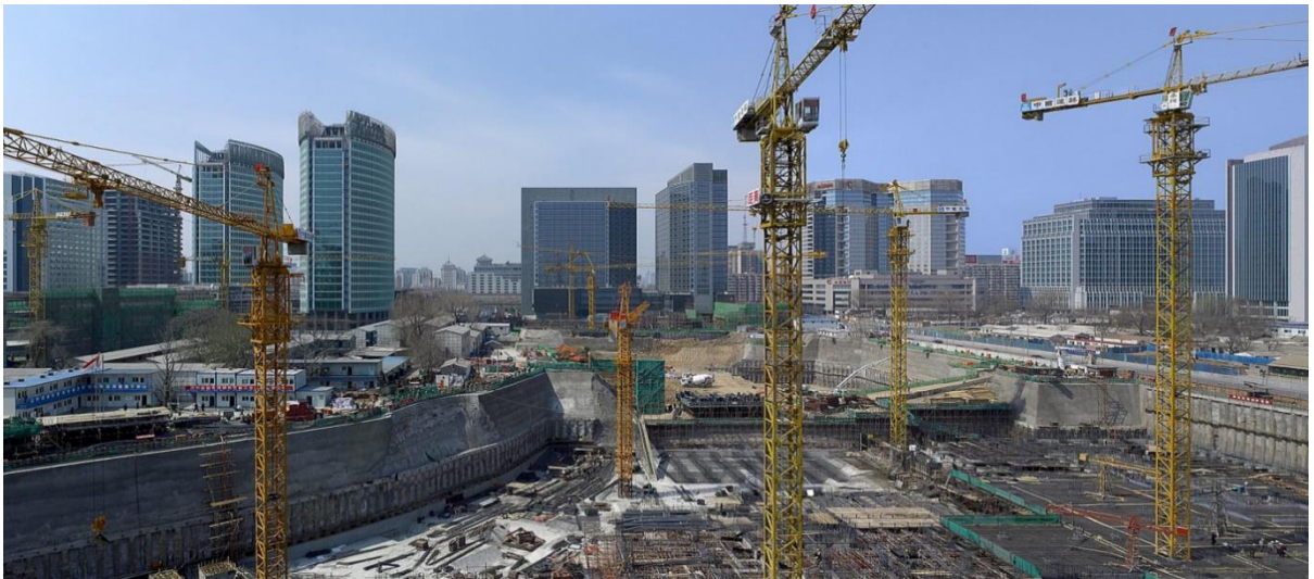
Figure 12: The Beijing Financial Street Centre-Piece Under Construction 41
