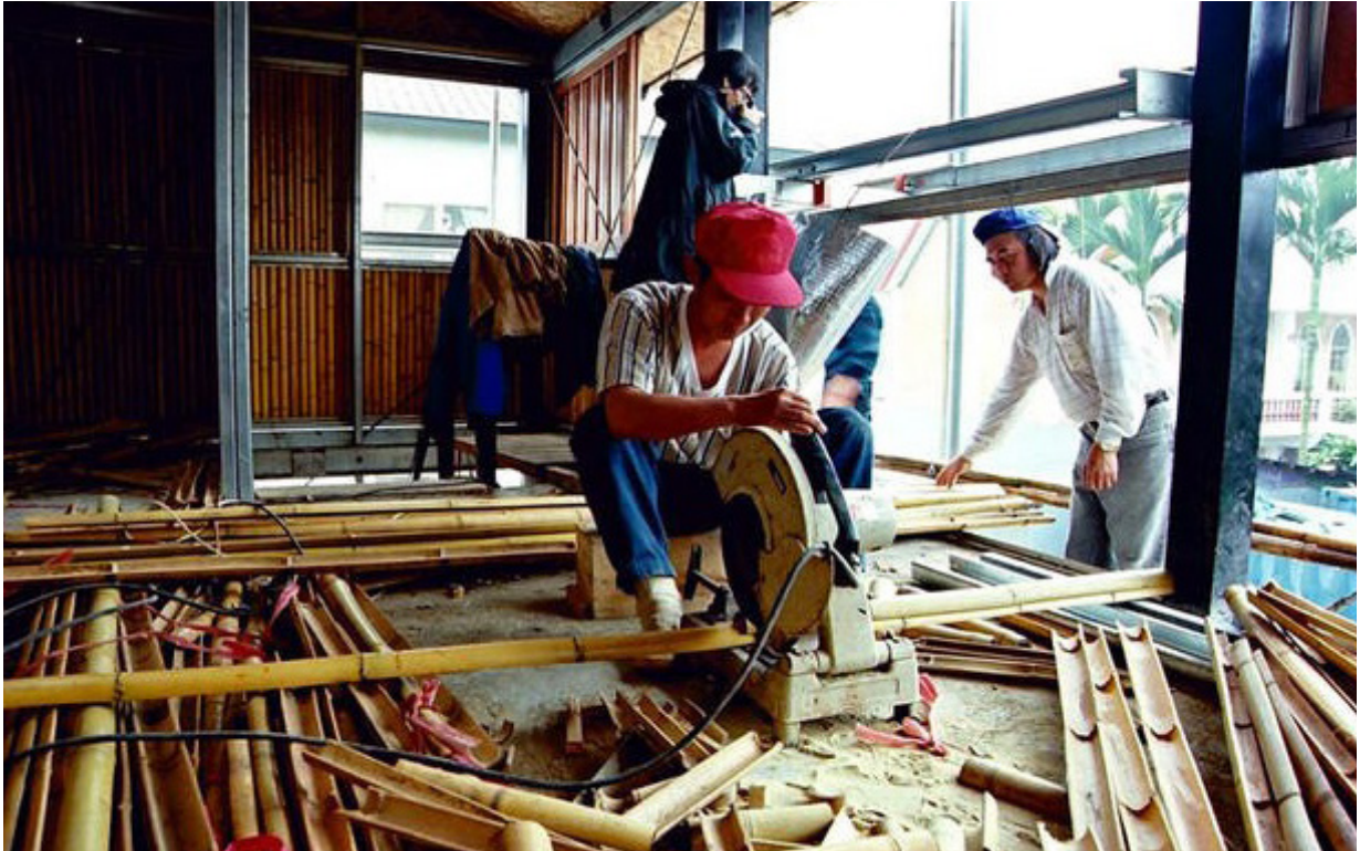
Fig. 1.8 Atelier-3's disaster-relief construction.
