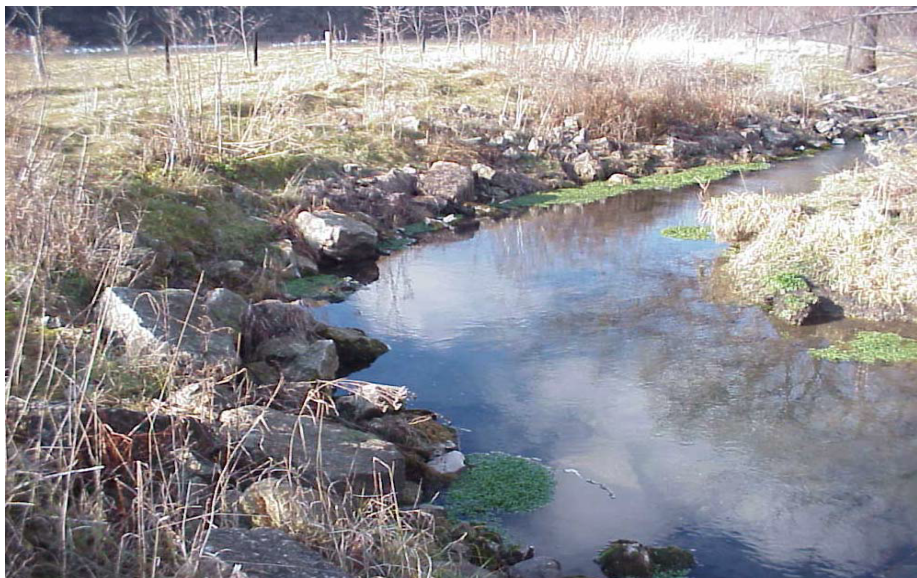
Figure 2: Large particles placed on the outside of a channel bend for erosion protection. These particles have been integrated with vegetation for further stability (IOWA Department of Natural Resources, 2006).
