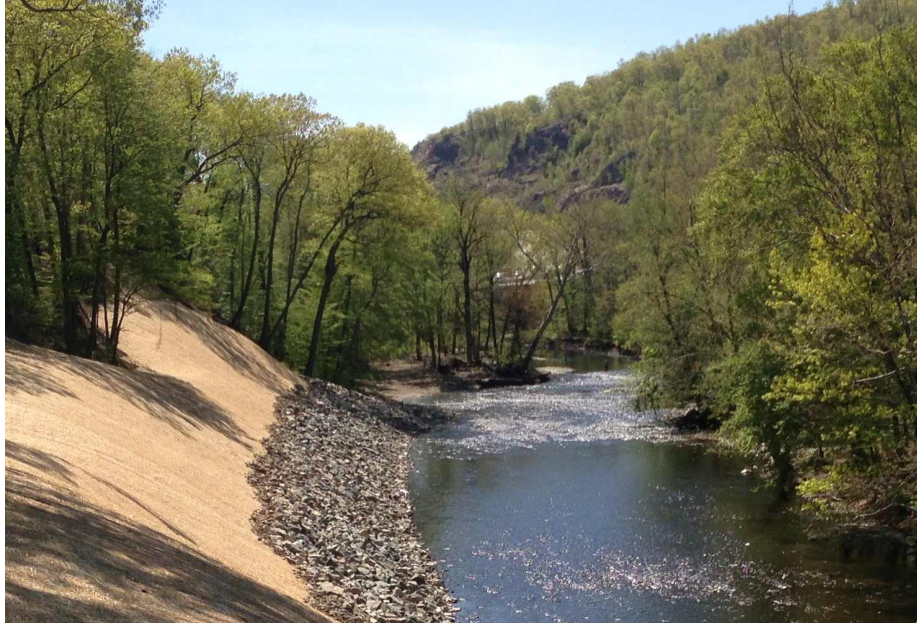
Figure 3: This photo shows the placement of riprap material on a channel bank for erosion protection (New Jersey State Soil Conservation Committee, 2014).
