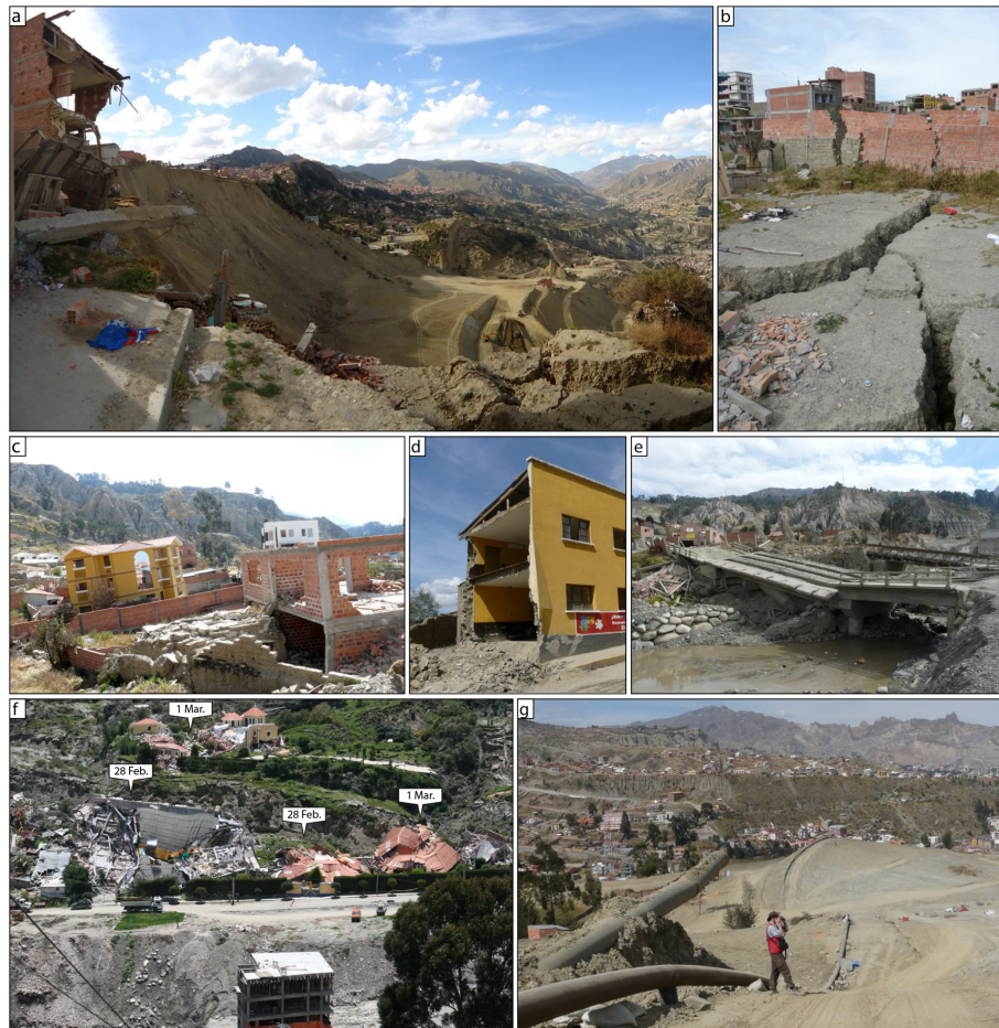
Figure 6. Impacts of the 2011 Pampahasi landslide. (a) Head scarp (80 m height) along the east margin of Pampahasi Plateau (note excavator and trucks in lower middle ground for scale). (b) Ground fissures in the northern part of the lower landslide mass. The wall in the background is \sim 2 m high. (c) Back-tilted houses and apartment buildings on the northern part of the lower landslide mass (movement was from left to right). (d) Community building with collapsed wall on the northern part of the lower landslide mass. (e) Bridge across Río Irpavi that was deformed and shifted from its footings on 27 February near the centre of the landslide toe. (f) Buildings on the southern part of the toe of the landslide that collapsed on 28 February and 1 March (dates of collapse shown; photo by Marco-Antonio Guzmán, 2 March 2011). (g) Water service line ruptured by the landslide (upper pipe) and replacement water service line (lower pipe). See Figs. 2b and 8c, d for locations of photographs. Photos taken by Nicholas J. Roberts in May 2011 unless otherwise indicated.
