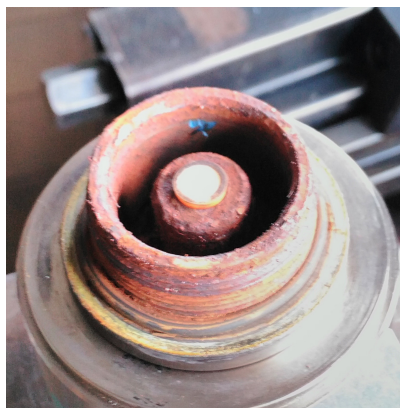
(a) Corrosion in the original valve which was attributed to nitric acid.
