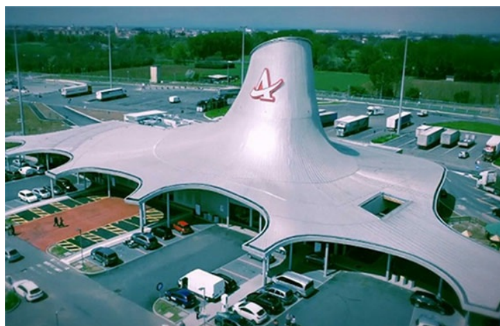
Figure 1 Villoresi East Autogrill structure
