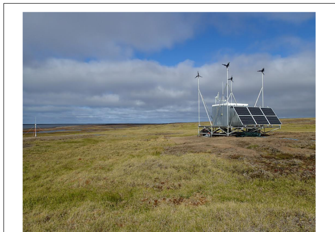
FIGURE 1 | Picture of an Arctic HF radar installation to the left and its corresponding remote power module (RPM) shown to the right. (Photo credit: Hank Statscewich, UAF, AK).
