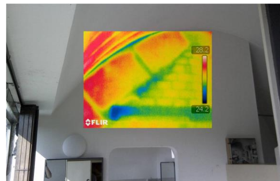
Figure 4. © A-BIME: Infrared camera picture: structure of the bedroom wall
