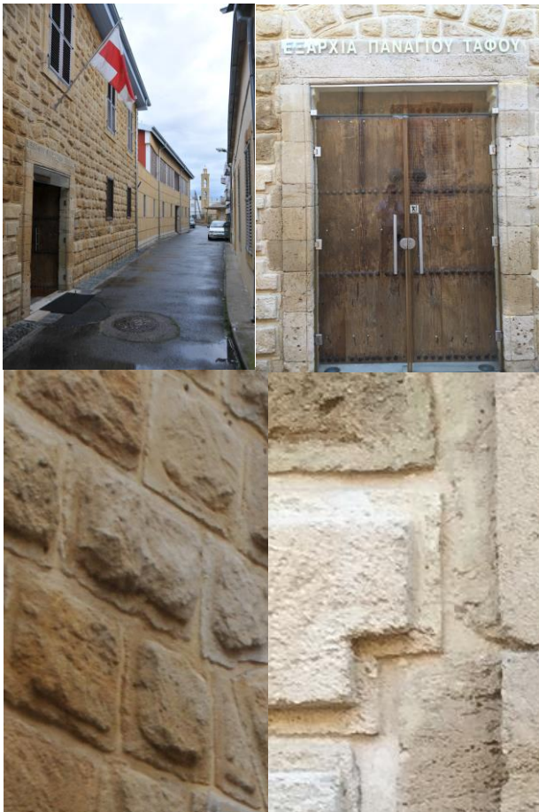
Figure 9. Repositories of materials and masonry arrangements: the Nicosia's Patriarchate external wall
