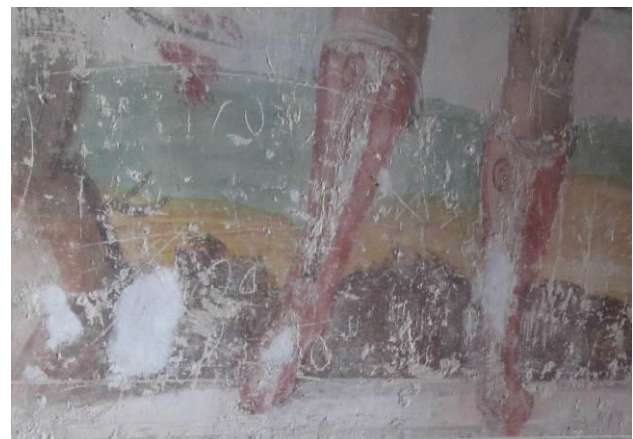
Figure 15: Wall paintings decay, room 4.
