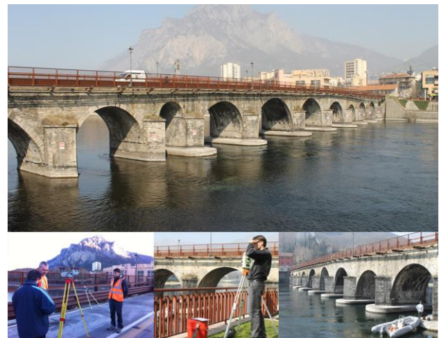
Figure 1. Azzone Visconti bridge and the 3D survey and levelling campaigns
