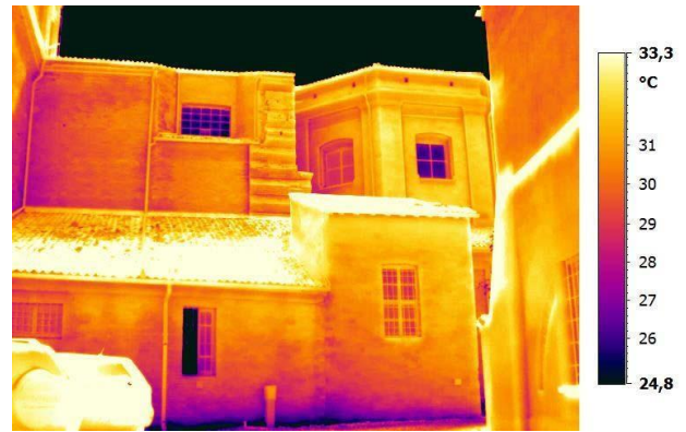
Figure 4. Mantua Duomo. Visible light and Thermogram (24 May 2017) of the North-East façade.
