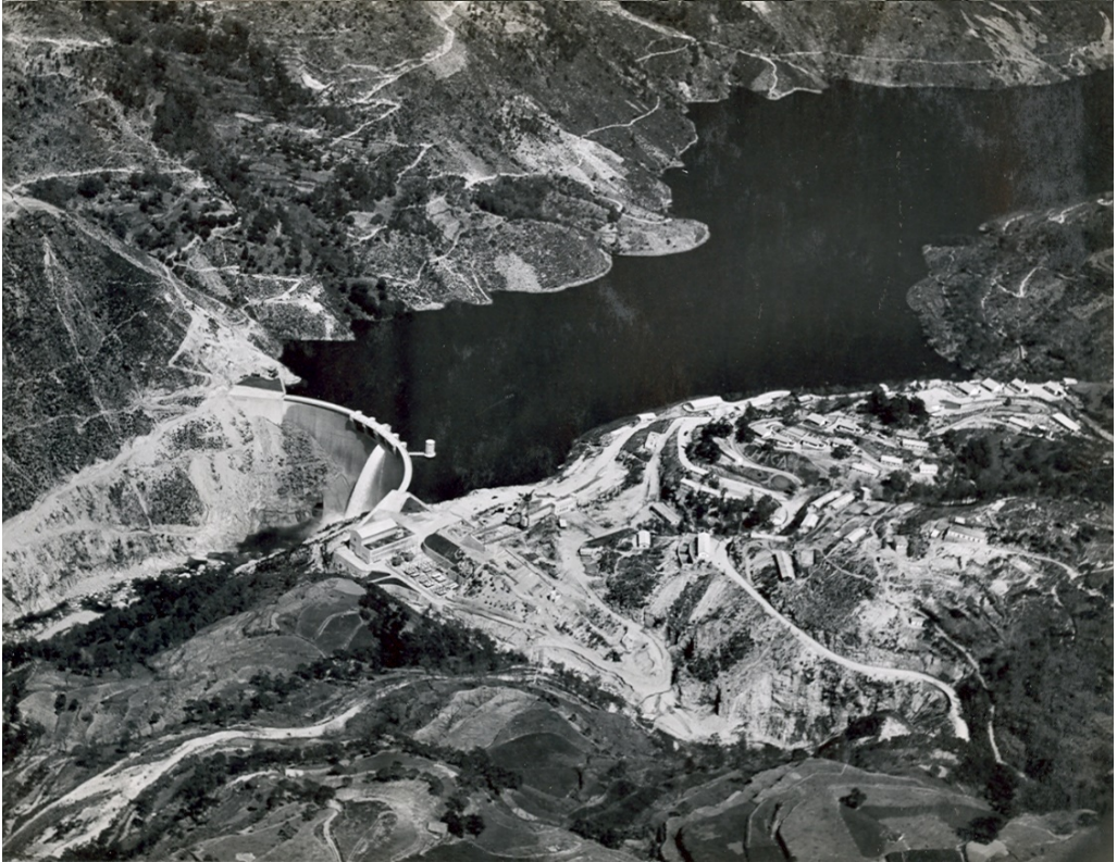
Fig. 2. Dam construction, Salomonde, 1955. Photo: Casa Alvão; Source: ATEDP.
