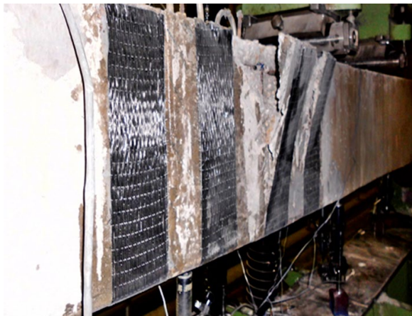
Figure 4. Delamination of concrete cover failure mode (B20-200S)
