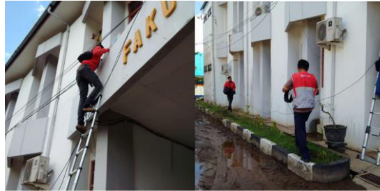
Fig. 5. Cable installation process
