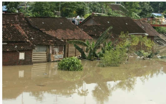
Fig. 4 Condition of Residential Area along River Bank Area of Bengawan Solo River Photo Author: Surakarta Government 2008
