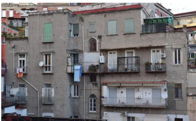
Figure 7: Typical pre-18th century apartment house, with completely unplastered facades
