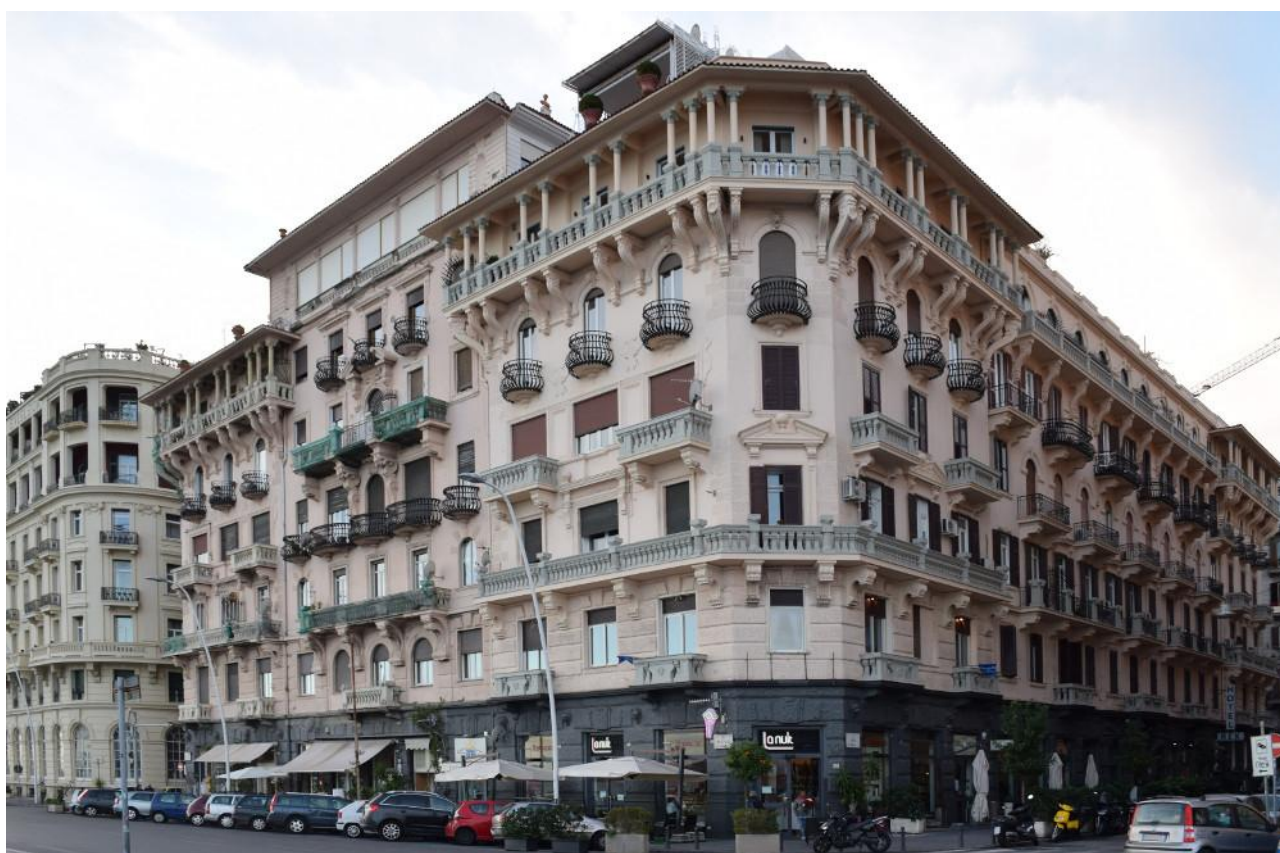
Figure 8: 18th-19th century building constructed on the Colmata di Santa Lucia
