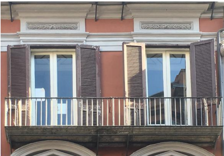
Figure 13: Balconies built with heavy piperno slabs supported by metal frames
