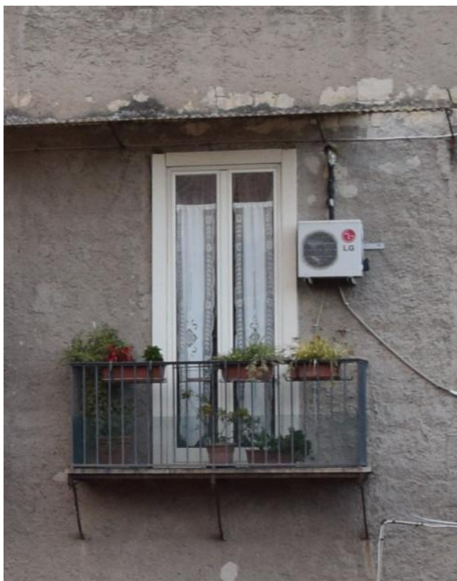
Figure 9: Balconies built with thin marble slabs supported by metal frames
