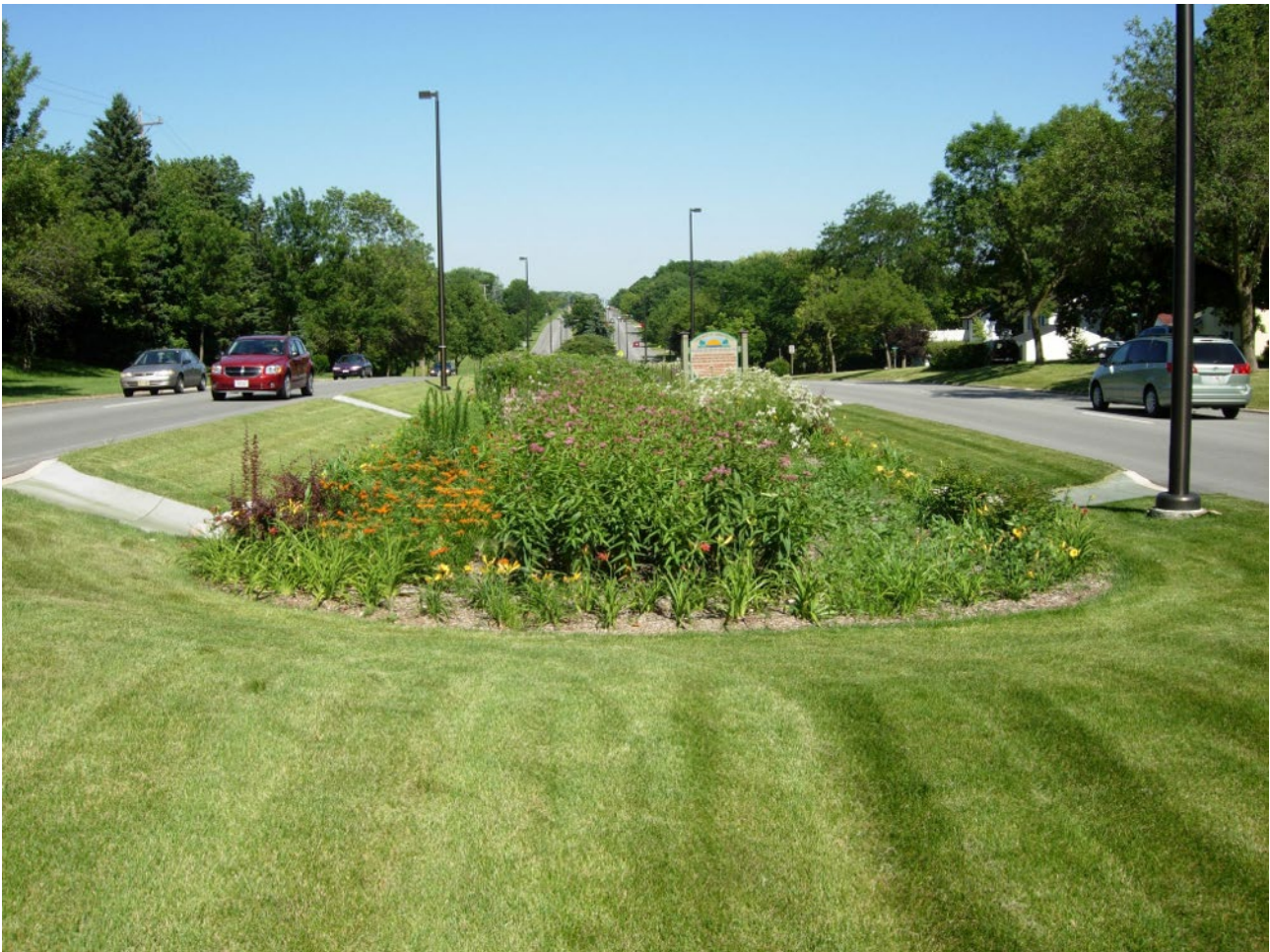
Figure 4: Bioretention / sideswale in median of Grange Avenue in Greendale, Wisconsin. Photos taken July 2010. Source: Aaron Volkening [CC BY 2.0]. Retrieved from Flickr.com
