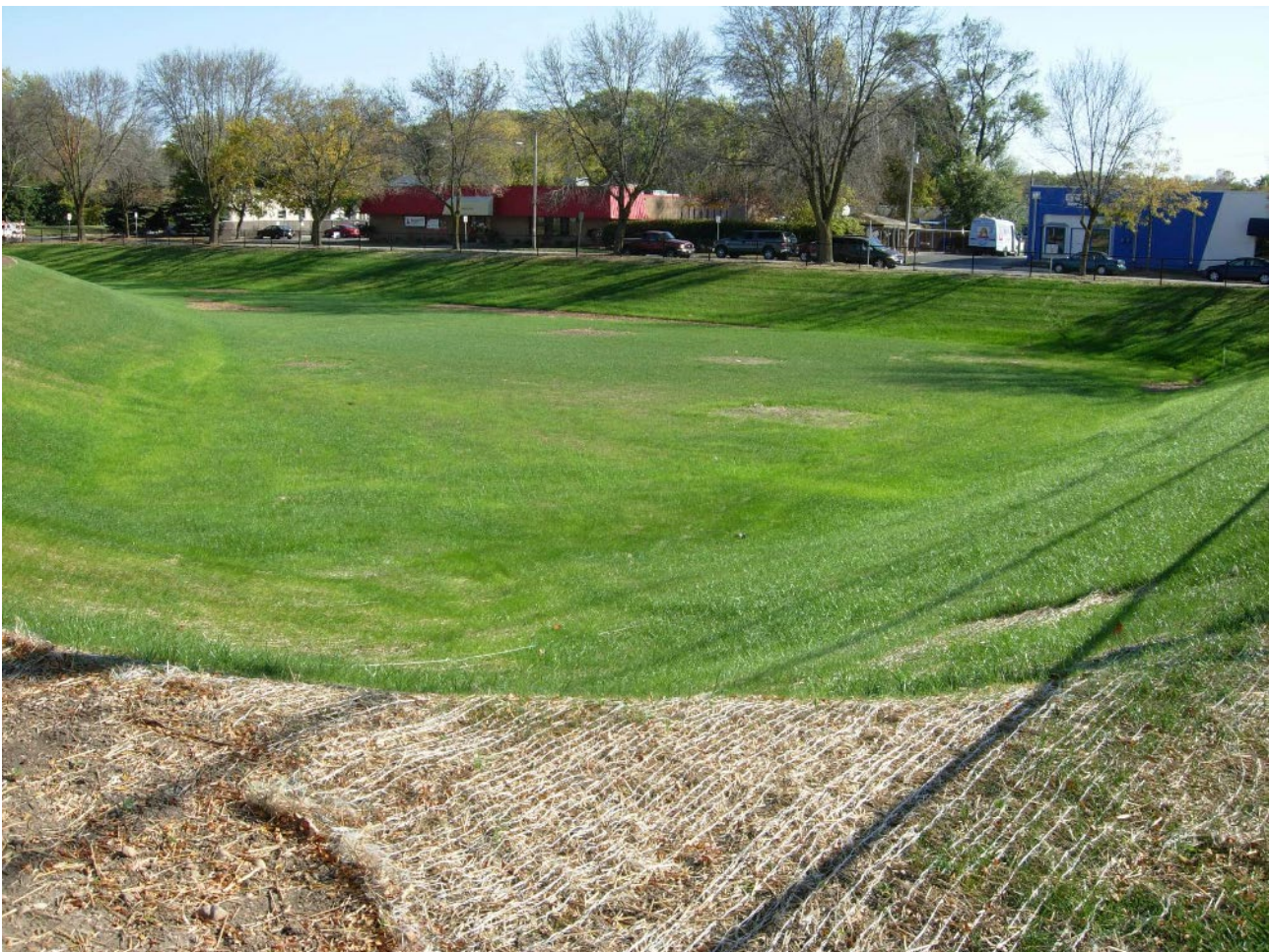
Figure 5: Dry stormwater detention basin in Grandview Park, Waukesha, Wisconsin. Photos taken October 2010. Source: Aaron Volkening [CC BY 2.0]. Retrieved from Flickr.com
