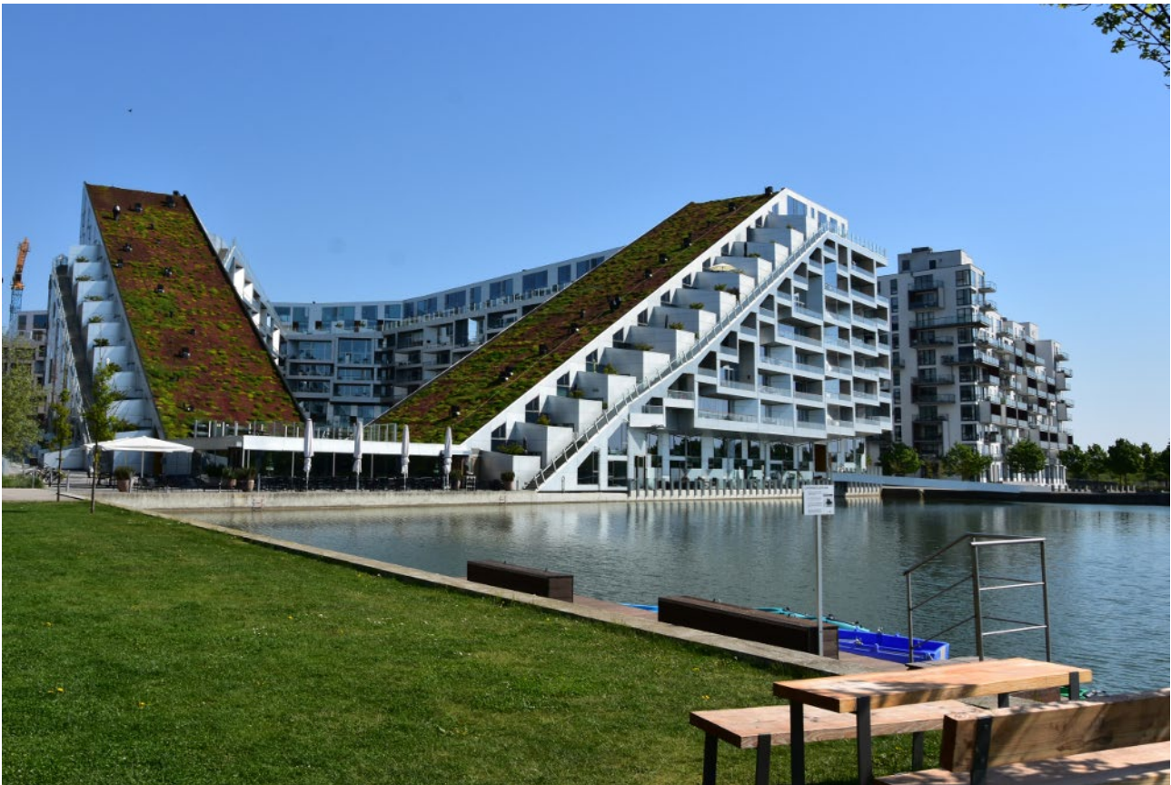
Figure 5: Green roof in the developing city area Ørestad, Copenhagen, Denmark. Source: image courtesy of S. Barbato, 2018.
