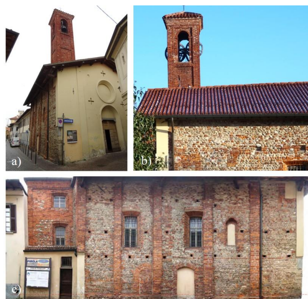
Figure 2. St. Antonio Oratory: a) the façade; b) the bell tower and c) the rectified north side with its stratifications.
