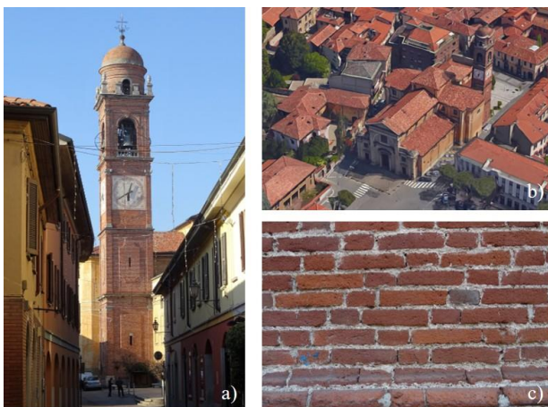
Figure 4. The Sanctuary of the Holy Virgin of the Rosary: a) the bell-tower; b) a sky view of the church and c) its masonry.
