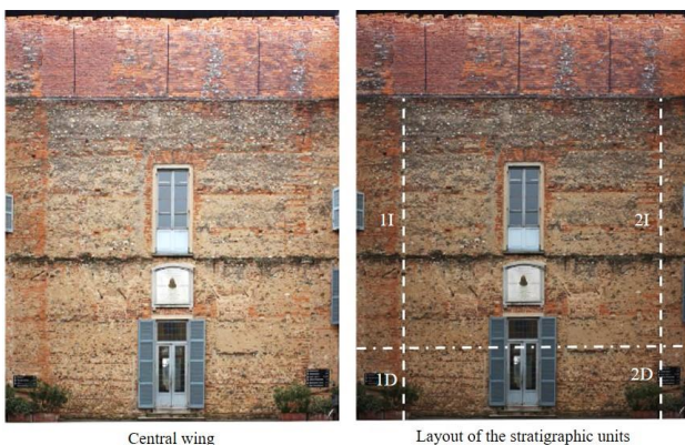
Figure 13. Localization of sampling areas in Palazzo Trotti, Courtyard façade, according to USM (1 and 2) and Direct (D) and Indirect (I) measurements.
