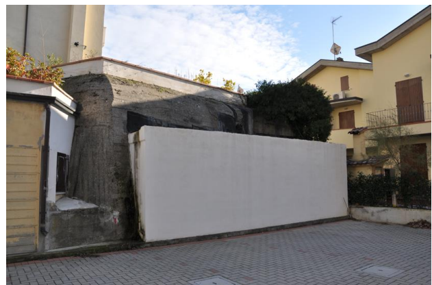
Figure 3. Lido di Savio (RA), Example of a bunker embedded in contemporary buildings. © Zampini, 2018.
