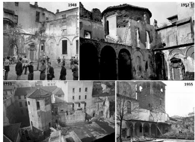
Figure 3. The transformations of cloister of the Monastery of St. Maurizio in the years following the Second World War.
