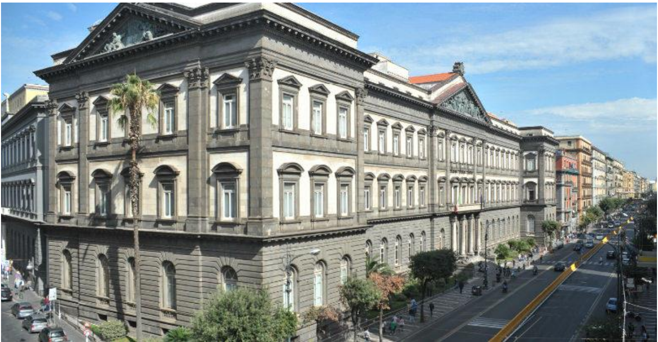
Figure 2. Naples. The front of the Federico II building on corso Umberto I (2016)
