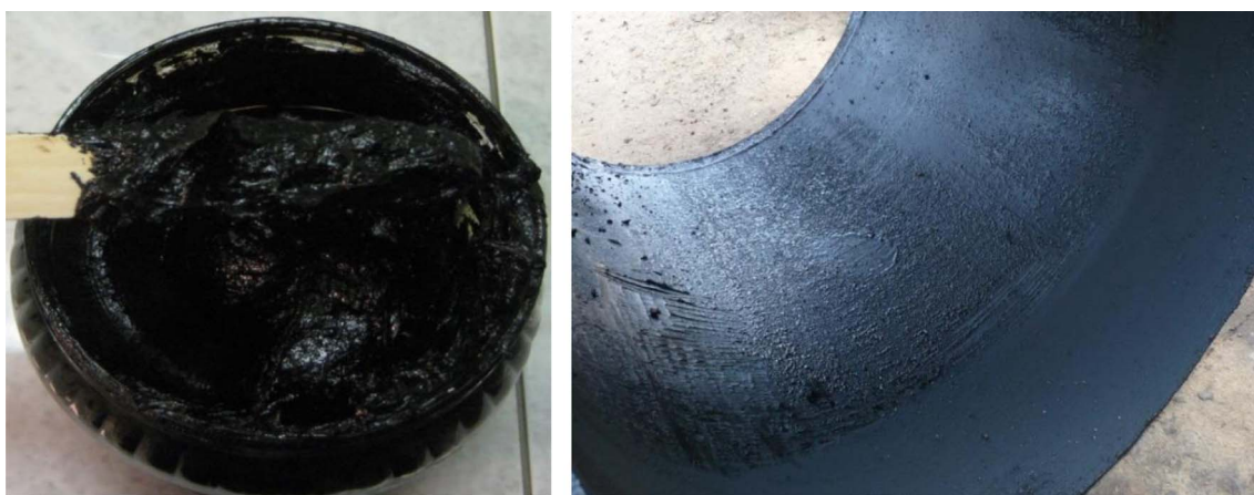
Fig. 2. Asphaltene-resin-paraffin deposits on the inner surface of the pipeline sample.
