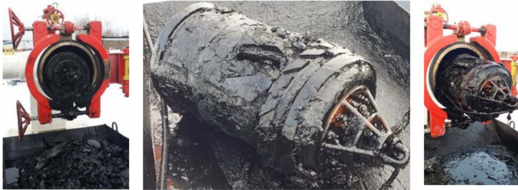
Fig. 6. Asphaltene-resin-paraffin deposit removal with mechanical cleaning units.
