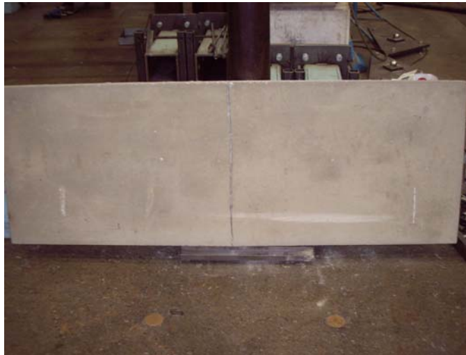
(b) Single crack in UR6
