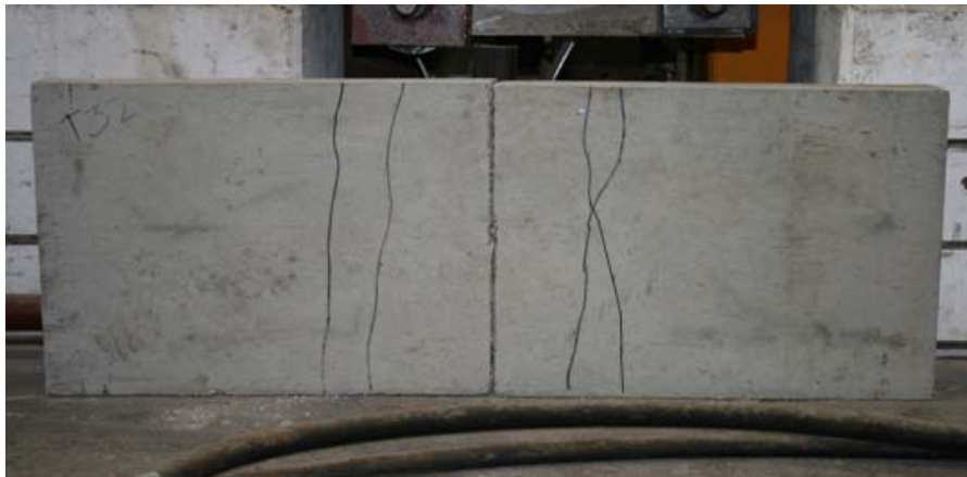
(b) Crack pattern
