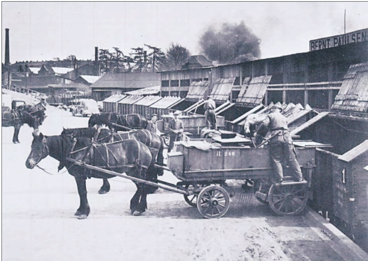
Figure 1. This photograph captures a part of the hygienic conditions in Oslo as late as in the years 1945-50: Waggons with human waste from the old fashioned bin or bucket toilets are emptied to be used for agriculture fertilization. This system, based on countryside traditions, was a hygienic misery when transferred to a crowded city, and it was gradually replaced by modern WC's in all houses. Normally, society and life conditions change at a slow pace and are hardly noticed in everyday life. But in an individual life span perspective, such transformations in many fields may be quite profound and are important for the assessment of earlier health exposure and for the understanding of the historical developments in morbidity and in public health approach as well. (Photo by an unknown photographer. Oslo City archive OB.X1643.)
