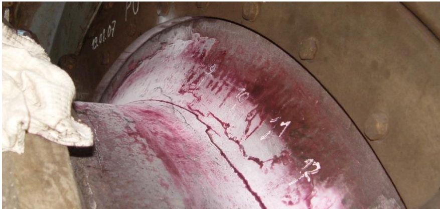
Fig.1. General view of cracks initiated from on transition radius and meshing on hydro turbine shaft
