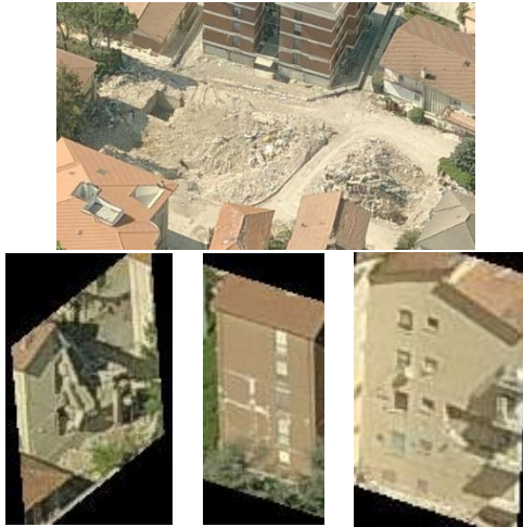
Figure 1. Top: example of two completely collapsed buildings. Below: examples of extracted façades. Left, partially collapsed building. Right and centre, two damaged façades with spalling and other damages while the facade is still standing
