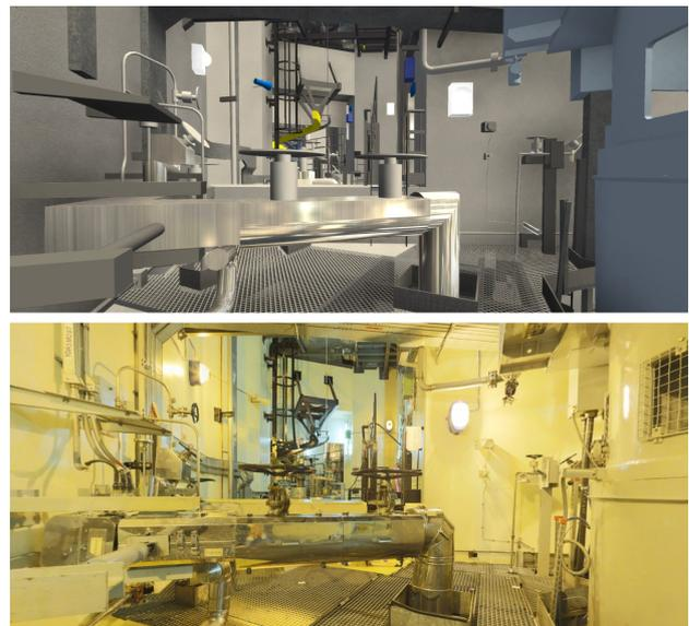
Figure 3. Data source: as-built 3D model and panoramic image accurately positioned and oriented.
