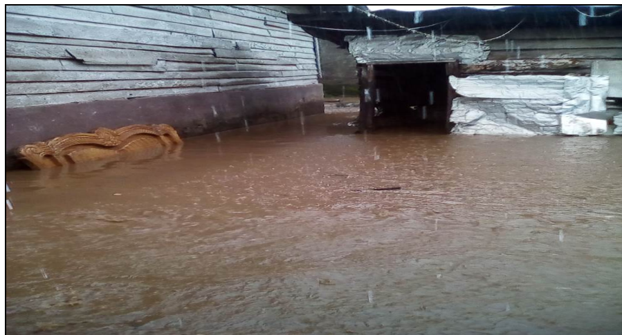
Figure 5.18 A photograph showing a flooded woodshop due to lack of a proper drainage system
