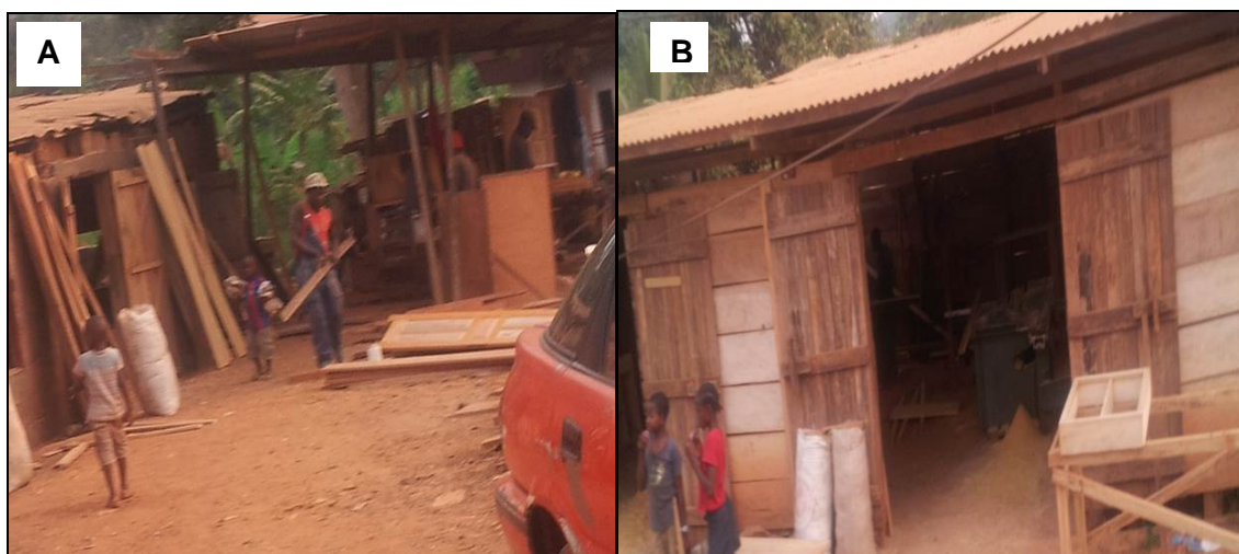
Figure 5.10 A photograph showing a roof-only workshop without side walls (A) and an enclosed workshop (B) with side walls constructed from wood
