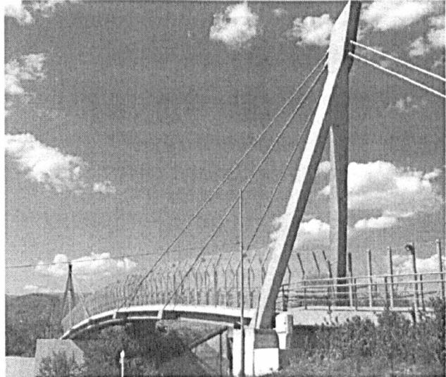
Figure 1.2: Footbridge in Sienna, Italy
