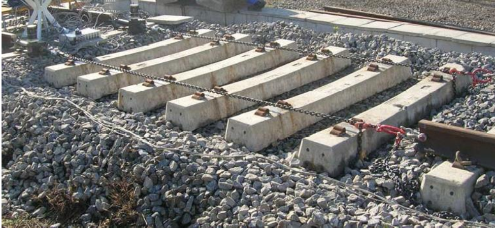
Figure 11. Second longitudinal pull test: detail of actuators linkage to the short track panel.
