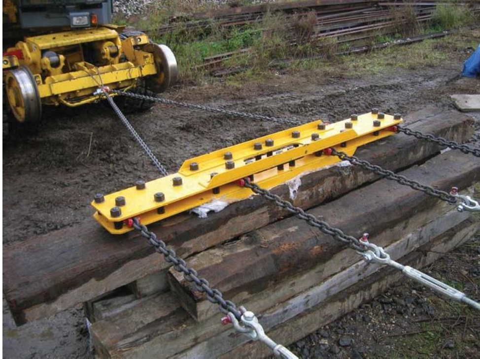
Figure 4. Loads transferring structure hooked to a railroad loader. FIGURE #4 219x164mm (300 x 300 DPI)
