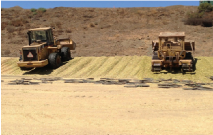
Figure 4. Packing the forage surface with the loader or crawler.
