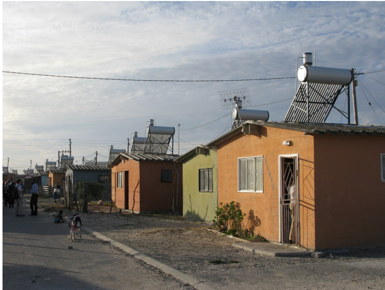
Houses fitted with solar water heaters by the Kuyasa CDM Project
