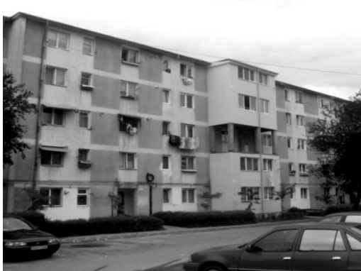
Low-comfort blocks: attaching new balconies
