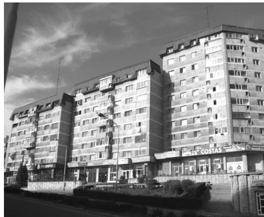
The 1980s: Blocks in prefabricated concrete panels
