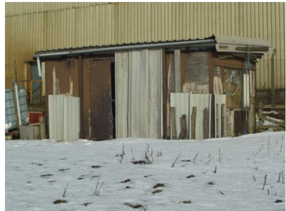
Plate 2:11c Shed repaired after use by Orlando for head-rubbing
