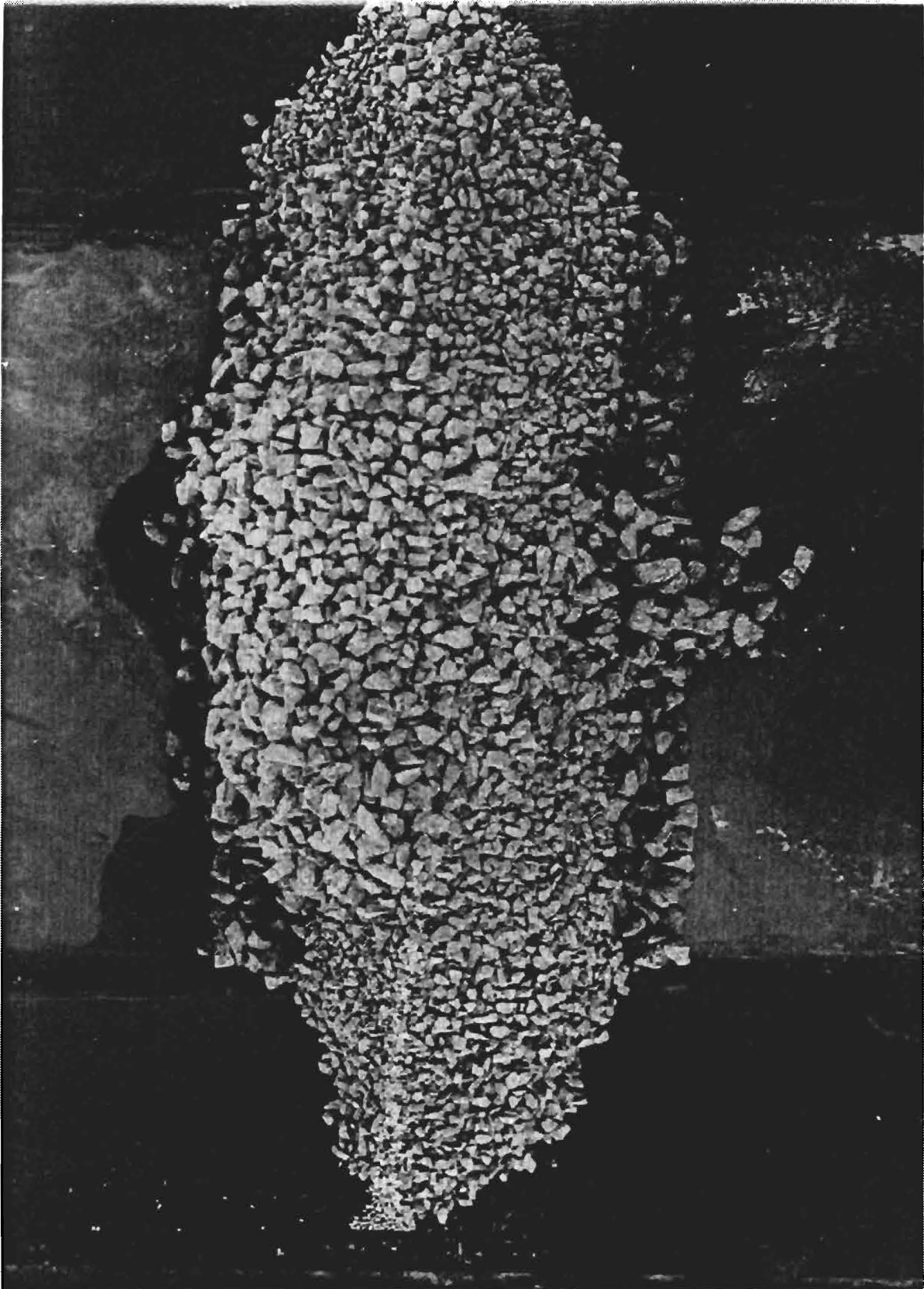
Fig. 27-Overhead View of Final Closure Dam (Upstream on Left Side)
