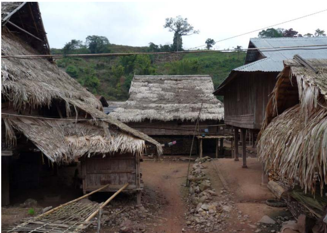
Picture 3. Electricity cables from pico hydro in an off-grid village in Phongsaly.
