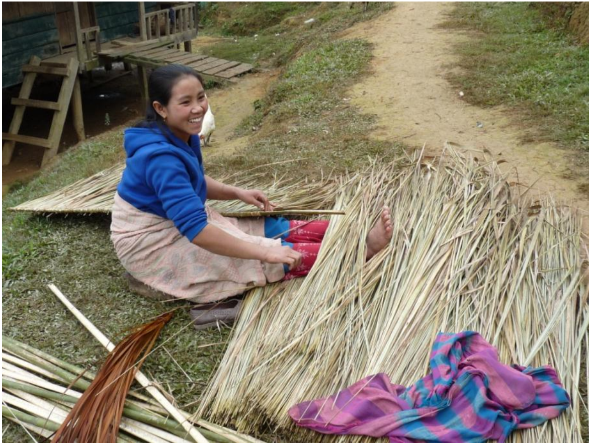
Picture 10. A woman in Houay Eouang village in Huaphan Province making a grass roof.
