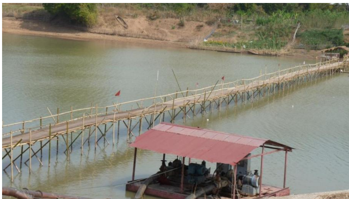
Picture 8. Irrigation pump at the Xedon River in Showvanakhiri, Champasak Province.
