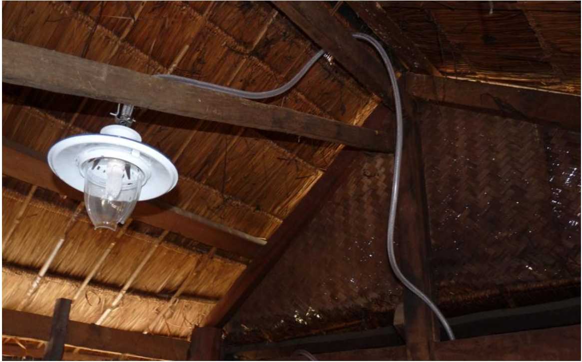
Picture 5. A light bulb in Vangkaben village running with energy from bio gas.
