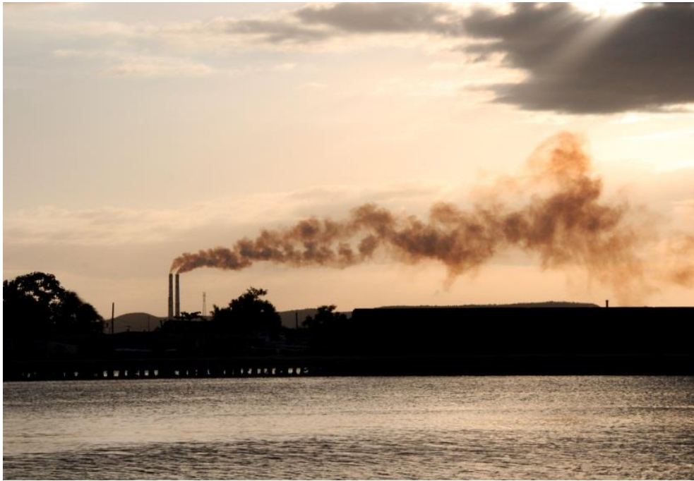
Picture 1. Old thermoelectric power plant in Santiago de Cuba.
