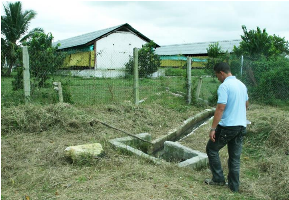
Picture 4. Biogas plant at a pig farm.
