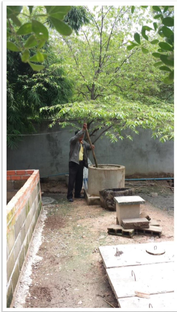
Picture 3 Feeding the input into a biogas digester in Cambodia, © Visa Tuominen
