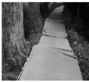
50-25% in Good Condition
