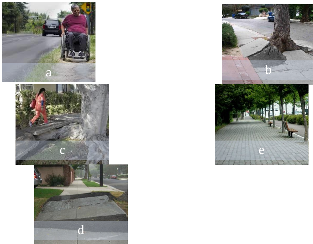
Figure 15 Percent of Sidewalk Usability; (clockwise from top left) a. Unpaved 48 , b. <25% 49 , c. <50% 50 , d. <75% 51 , e. 100% 52
