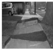
70-50% in Good Condition
