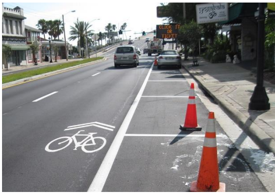
Markings of Bike Lane on a Road Segment
