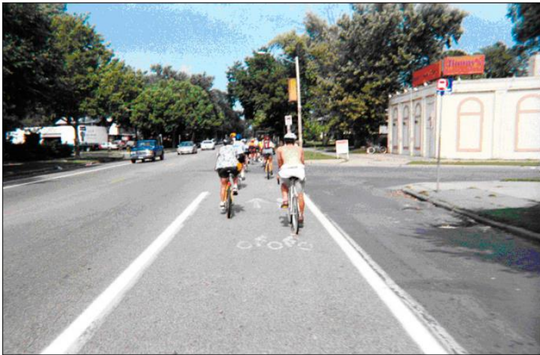
(b) Bike Lane on a Road with Curb but no Gutter 29
