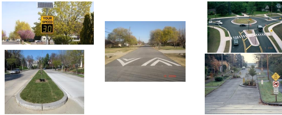
Figure 12 Traffic Calming techniques for road segment; (clockwise from top left) a. Speed enforcement 37 , b. speed bump 38 , c. roundabout 4 , d. chicane 39 , e. median 40
