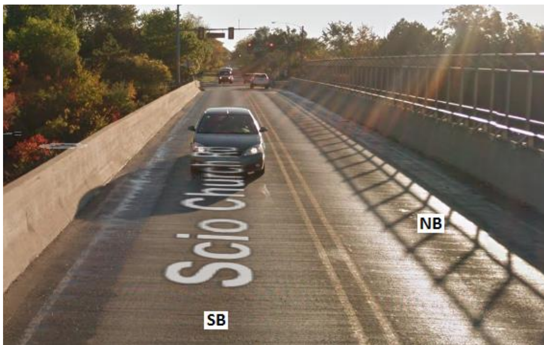
Figure 2-26. Scio Church Road bridge over I-94 (Source: Google maps)
