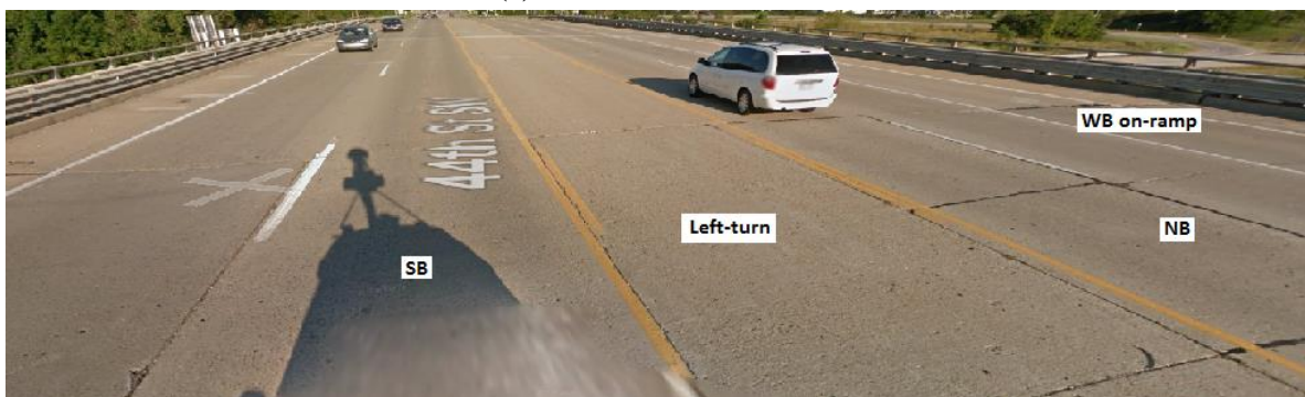
(b) A view of the bridge deck
