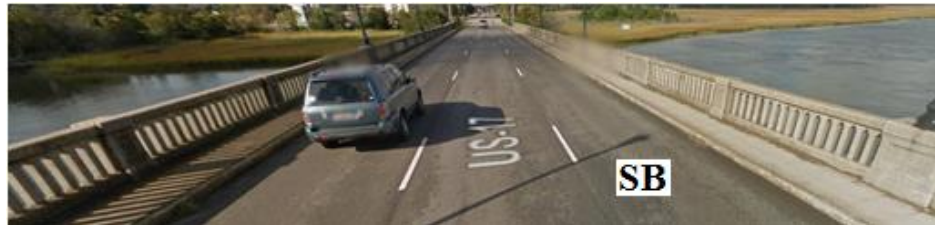
(b) Southbound bridge
