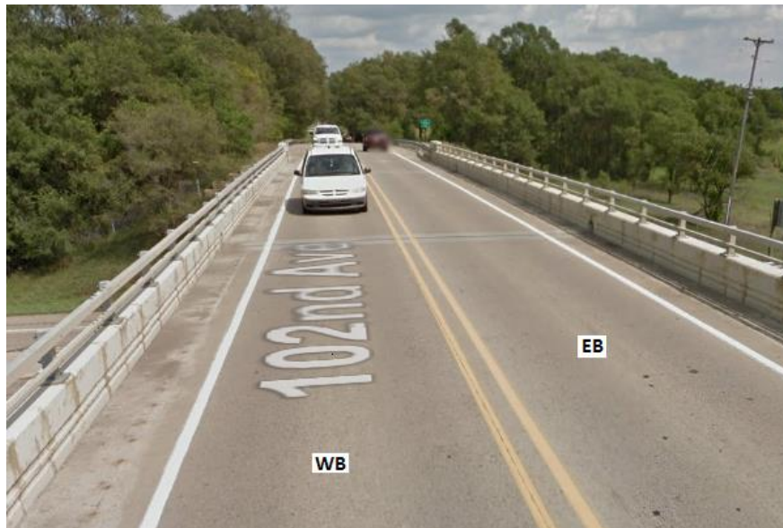
(b) A view of the bridge deck
