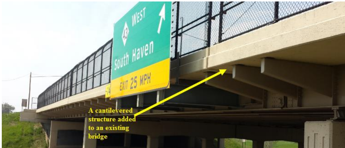
(a) Cantilevered structure
