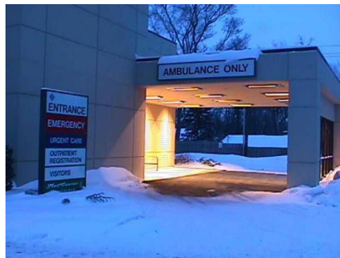
Figure 5-29. Infrared heaters implemented at a hospital (Source: MEHA 2015a)
