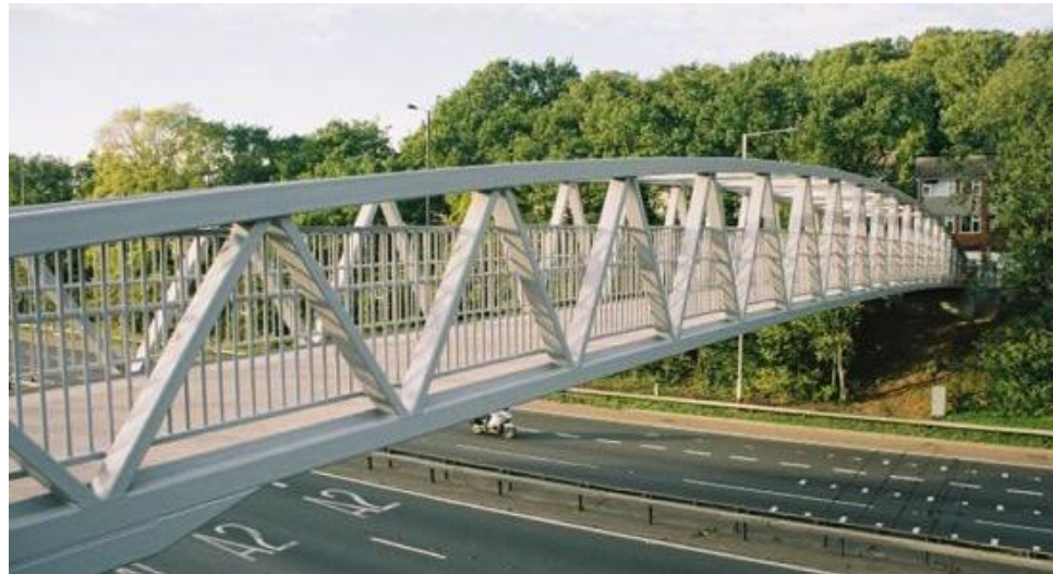
Figure 4-1. A bridge crossing a freeway (Source: Pinterest 2016)
