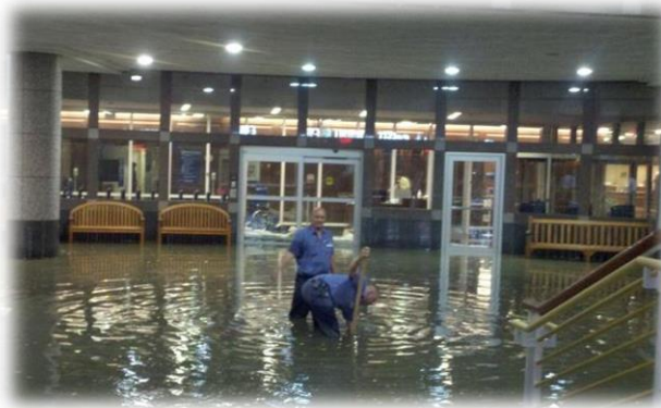
Figure 3-6. Flooding of the Rochester subway (Source: Sederstrom 2013)
