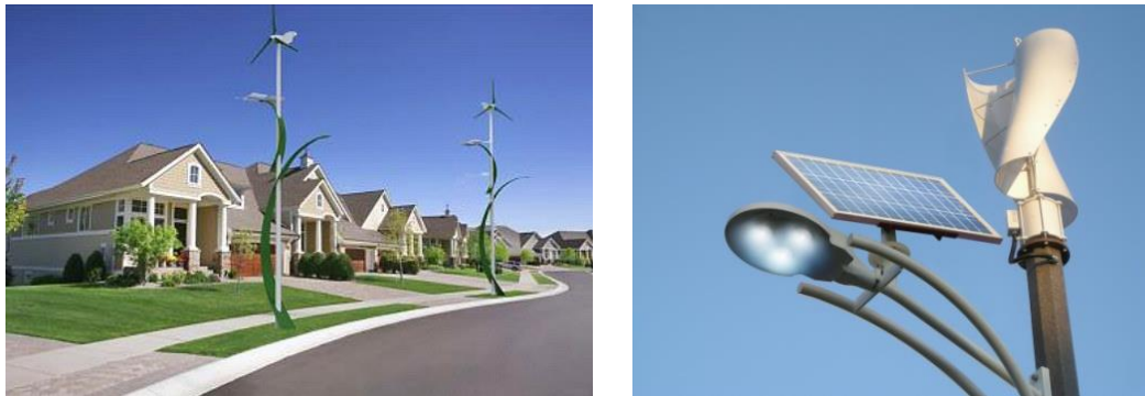
Figure 5-6. Wind-solar hybrid street lighting systems (Source: Sunning 2015)
